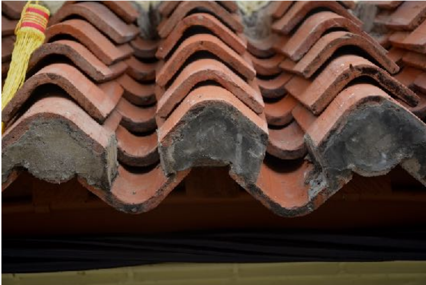
Photo 14: V-terracotta roof tiles of the new building observed from the South facade.
