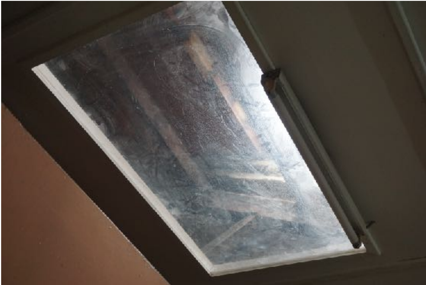
Photo 44: Plastic covered cutouts in the plasterboard ceiling of the first floor acts as skylights, transmitting daylight into the spaces.
